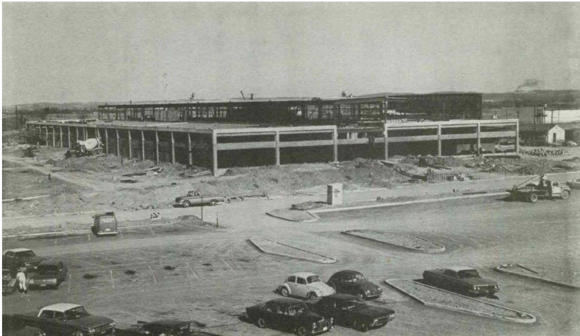
Figure 8 – USAMRIID Laboratories Building 1425 Under Construction - 1968 68
