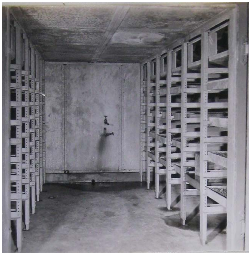
Figure 12 – View of the growth chamber– example from Crops Pathogen Pilot Plant 165 “View inside constant temperature cabinet arranged for shallow trays”
